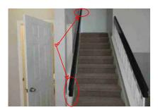
15.2 - The balusters in the stair rails are more than four-inches apart and are not child safe. Therefore, you may wish to add a protective barrier.
