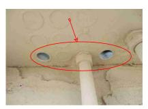
5.2 - The exterior panel cover latch is damaged, and should be serviced.
